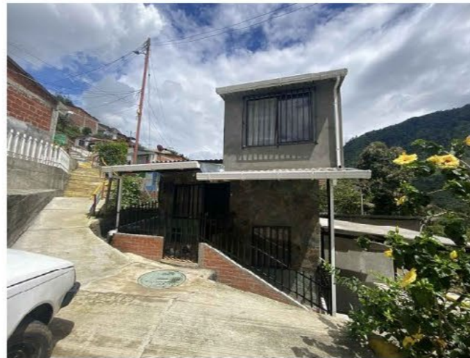
M40 | Cra 6a | Fachada 7-33.
